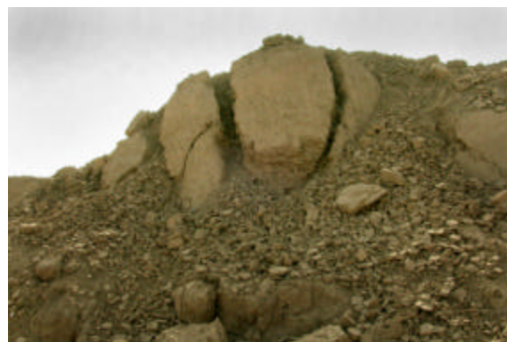
Figure 17: Collapsed round turret on the ramparts that shows evidence of having burst apart from collapse of internal layers.
