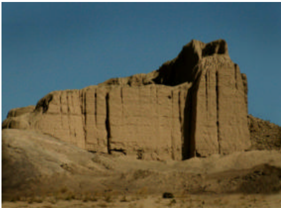
Figure 27: The unrestored Khale Dokhtar, a small Arg (or citadel) on the riverbank opposite the Arg-e Bam that survived the earthquake with the collapse of some arches. The high walls of the massive structure otherwise survived intact. (Termites and other insects were also in evidence where the collapses occurred.)
