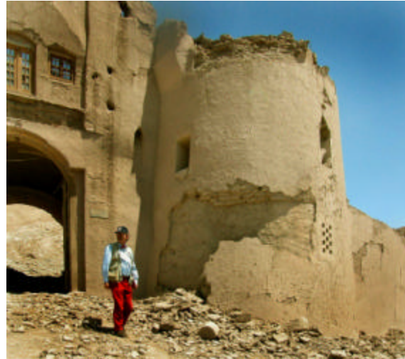
Figure 16: One of the few surviving turrets has evidence of timber reinforcement that extends through the walls, probably from a timber floor structure at the level just below the windows.
