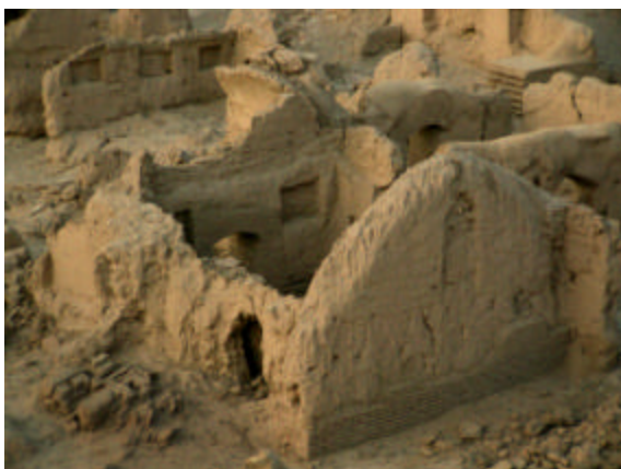
Figure 11: Unrestored ruins in the Konari neighborhood of the Arg-e Bam that survived the earthquake with comparatively little damage.
