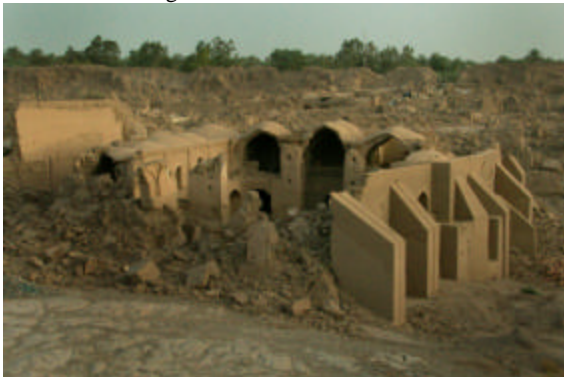
Figure 19: The ruins of the Caravansary show that the domed rooms on the second level behind the buttresses have collapsed, while the ones opposite still remain. There are no buttresses behind the external wall of the opposite side. The base of one buttress is crushed.
