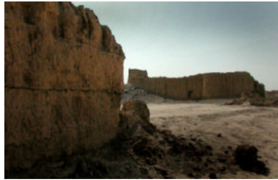
Figure 3: Unrestored ancient earthen structures just outside of the Arg walls to the north after the earthquake. These structures were only lightly damaged.
