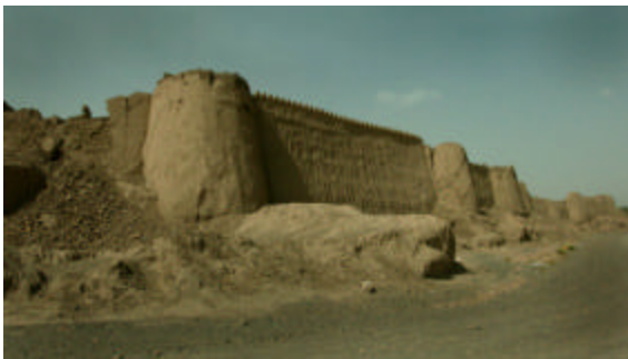
Figure 18: North-facing ramparts that were significantly less damaged in the earthquake than the other city walls. Notice that the crenellations are still intact on this one section, the only section where that was observed to be the case.
