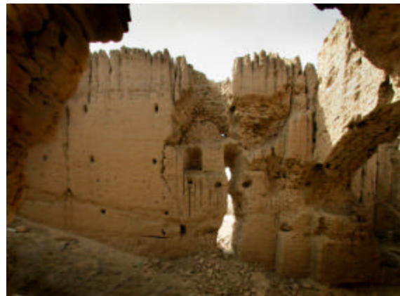
Figure 20: The interior of the unrestored structure in Figure 3 showing 3story high walls that survived the earthquake. Notice the older section with later work constructed around it. This is a good example of the onset of damage at the interface of construction of different age and type, as a small area of collapse has revealed this interface. Notice the debris on the ground.
