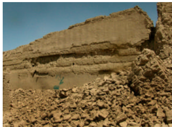
Figure 24: South-facing outside wall of the stables courtyard showing how the layering of the chineh walls has interrupted the cracking and collapse of sections of the wall, thus helping to maintain the stability of the partly undermined upper part of the wall.
