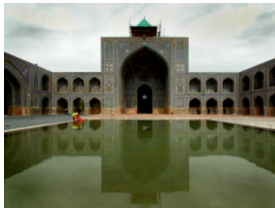
Figure 21: The Imam Mosque in Isfahan, April, 2004. The inner cores of many of these walls and the walls of other great monuments in Isfahan are constructed of unfired clay.
